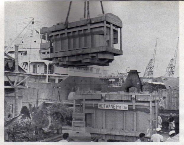
Unloading of Power Transformers at Bombay Docks — five such Transformers totalling about 50,000 KVA have been supplied to various grid sub-stations of the Chambal Hydel and Irrigation scheme in Madhya Pradesh.
