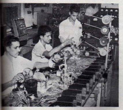
Testing of amplifiers, pre-amplifiers, etc., after assembly.
